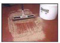
Sweep back and forth with a stiff brush until the spill is totally absorbed and the surface is free from any residue
